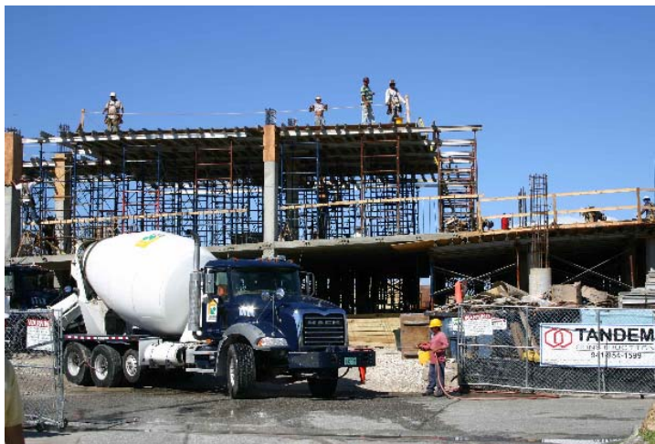
Hyatt Siesta Key Beach Construction Site August 2008
